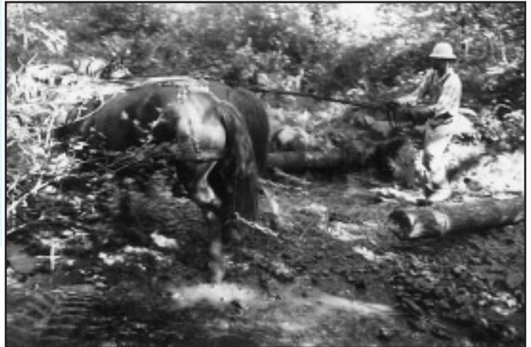
Figure 1. When it is necessary to work instream or beside the channel, draft horses causes relatively less physical disturbance of the streambed and banks.
