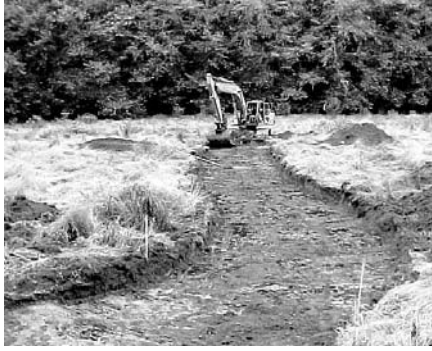
Figure 3. Construction of the new Karnowsky Creek channel, summer 2002. Stakes in foreground identify the location of a transition from a riffle to a pool. Note the excavated mounds of soil left on the floodplain.
