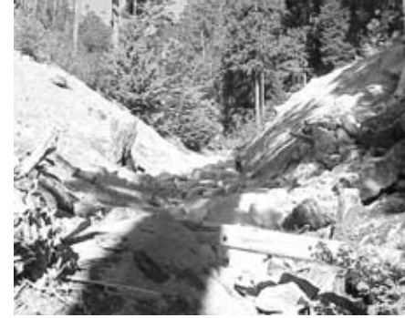
Major road fill after removal as part of decommissioning project. Fill removal allows reconnection of streams and significantly reduces future risk of wash and maintenance costs tied to major storm events.
