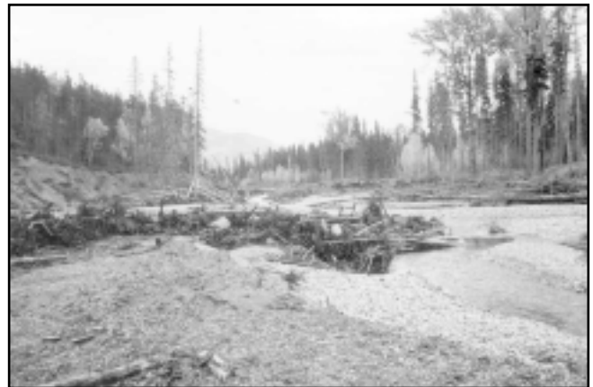
Figure 1. These huge logjams were constructed following removal and subsequent burning of logjams that were in place in Pine River during a Pembina Pipeline oilspill that occurred in August 2000. ▲
