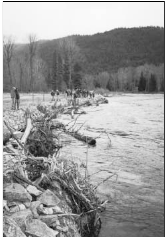
Participants at the BC - US Technical Exchange visiting a recent rip-rap and LWD treatment of an eroding bank at the West Kettle River near Beaverdell. (Work completed by Attrill Woodworking Services.)
