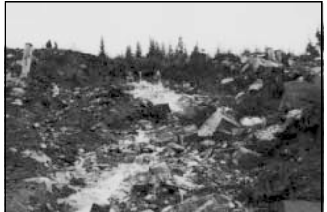
Figure 3. Photograph of the slide's initiation zone. Note the planar nature of failure surface, high cut tree stumps supporting road fill and abundance of water flowing over the headwall of the slide.
