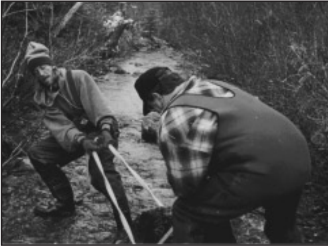
Figure 4. The boulders were placed on the rubber and the straps of the hand sling were pulled.
