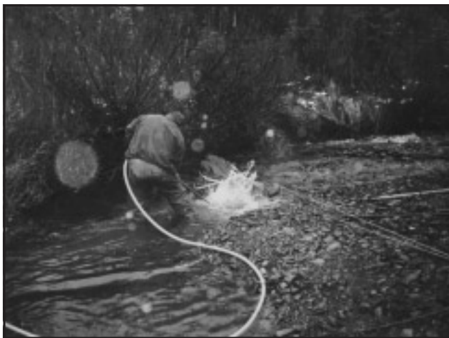
Figure 1. The hand wand with compressed air was pushed into the stream, creating air pressure to loosen the fine material around the boulders.
