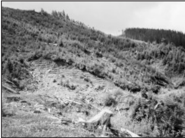
Figure 7. Modified brush layers used to stabilize the slope.
