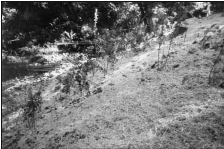
Figure 4. Base of rehabilitated slope, vegetation and Sediment-Lok™. Background shows restabilized stream channel.
