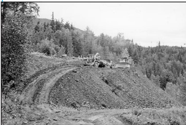
Figure 4. Conventional road stabilization, July 1996.
