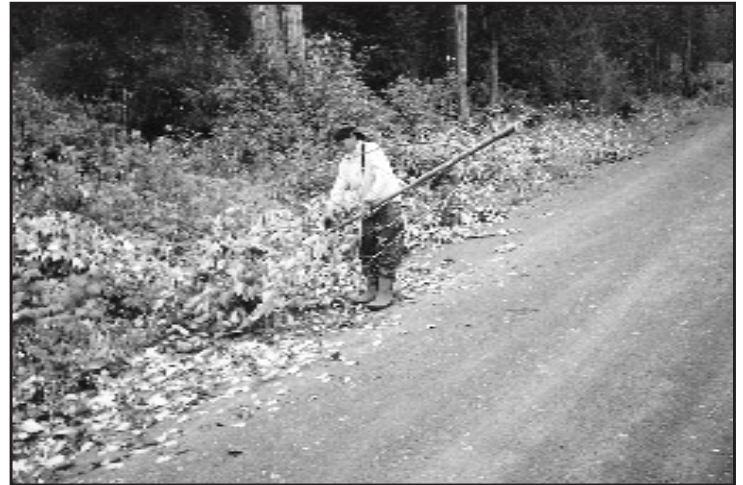
Figure 10. Forest worker preparing cuttings for live pole drain construction (from Rabnett 1997)
