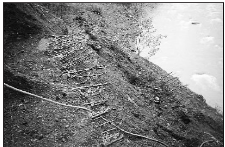
Figure 8. Three days of soaking ensures the success of sprouting. Root development is controlled by the soaking period, and is limited by the installation technique and site conditions (from Rabnett 1997).
