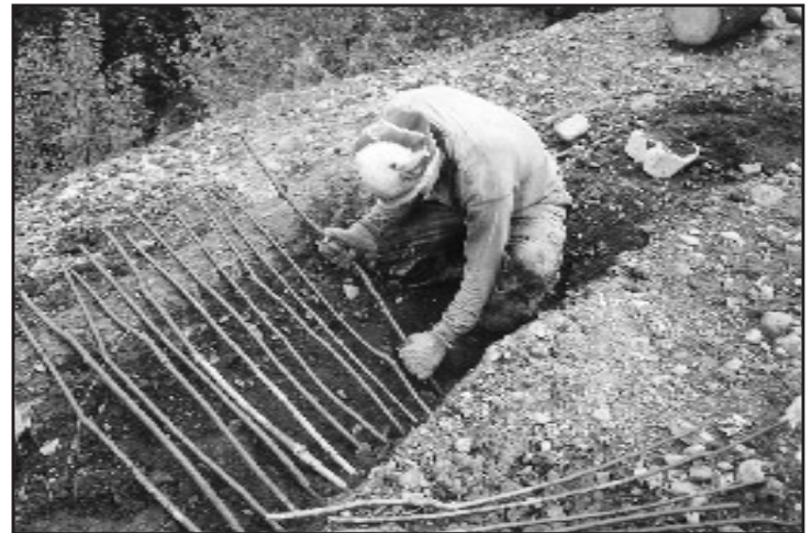
Figure 7. This forest worker is placing de-leafed, soaked, and sprouted cuttings in a modified brush layer (from Rabnett 1997).
