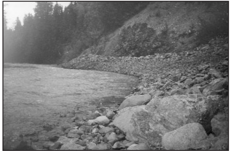
Figure 5. Finished berm constructed instream to prevent undercutting slopes.
