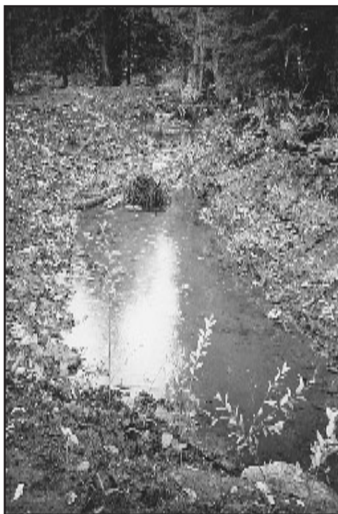
Figure 6. Channel construction provides both pool and riffle habitat.
