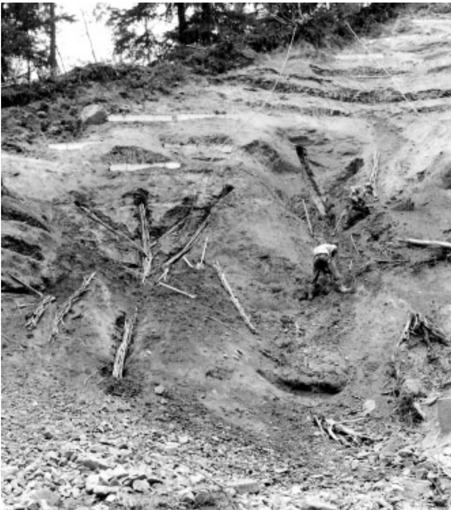
Figure 4. Site 1: Live pole drain installation.
