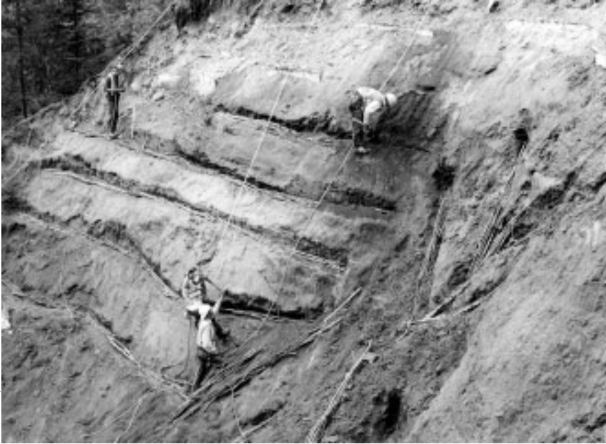
Figure 3. Contour facine installation.
