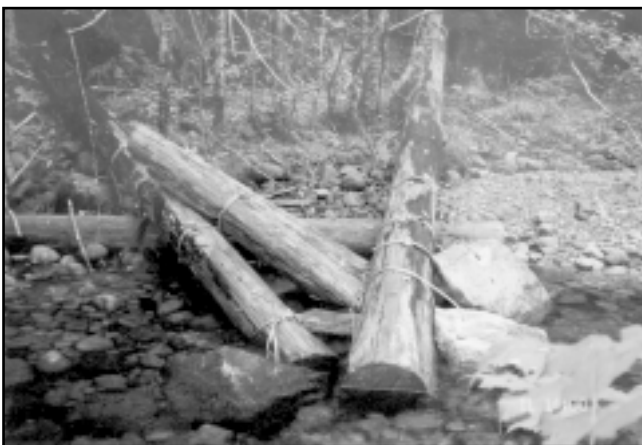
Figure 1. A LWD structure constructed by crew labour, supported by helicopter.
