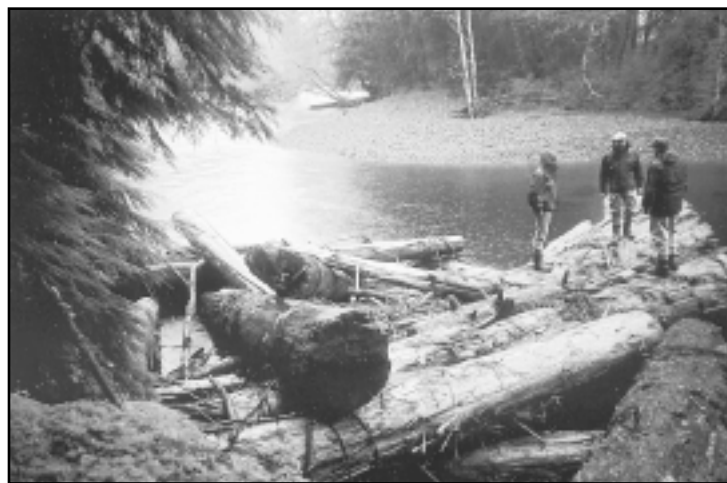
Inspecting a LWD structure on the Mahatta River.
