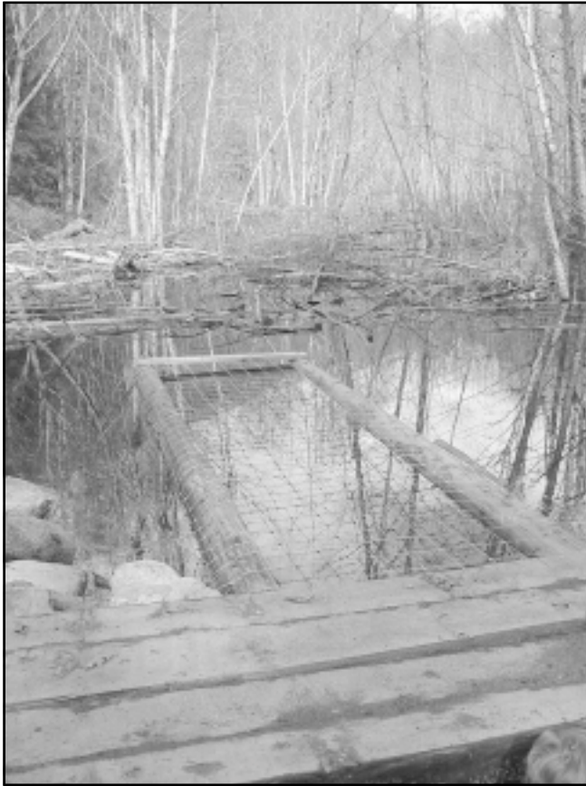
Figure 5. This beaver baffle helps deter movement of beavers back into the Bulbeard Creek ponds.
