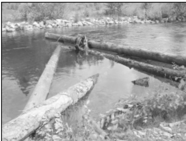
LWD structure creates habitat in Centennial Channel.
