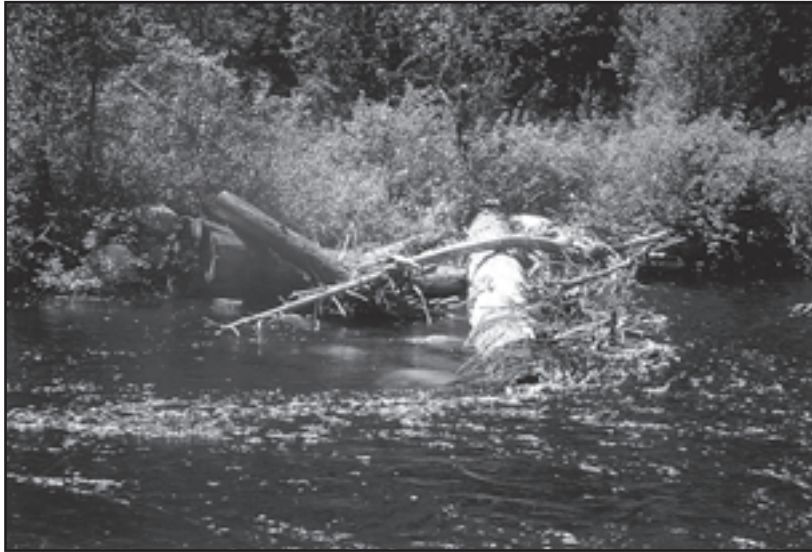
Figure 3. An example of a lateral triangular structure designed to collect driftwood and scour pool habitat for rainbow trout and mountain whitefish in the West Kettle River.
