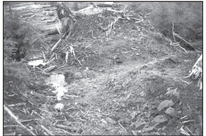
Figure 2. When a cross ditch has an inward slope, as shown here, the water cannot drain from the ditch.
