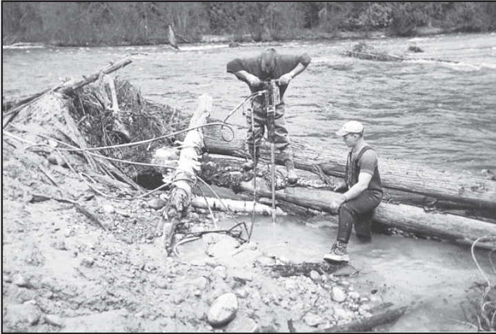
Figure 2. Installing the soil anchor with hydraulic jack in the Little Slokan River, Slokan Valley.
