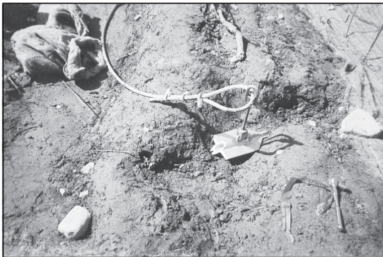
Figure 1. Manta Ray™ soil anchor with the cable attached.
