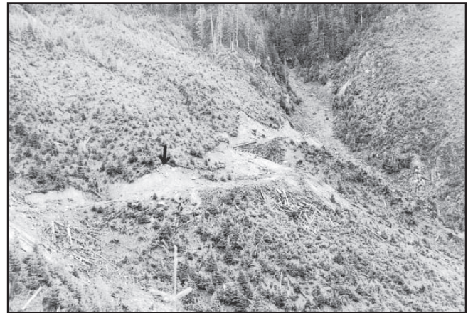
Figure 4. View of Misery Creek Watershed before road deactivation (Road number 400.)
