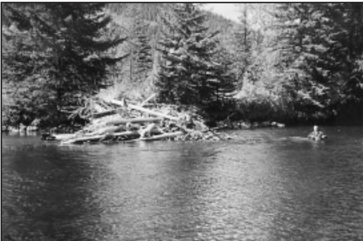
Figure 4. The same location as above, one year later. Note the extensive jam and the deep water, similar to natural lateral log jams.
