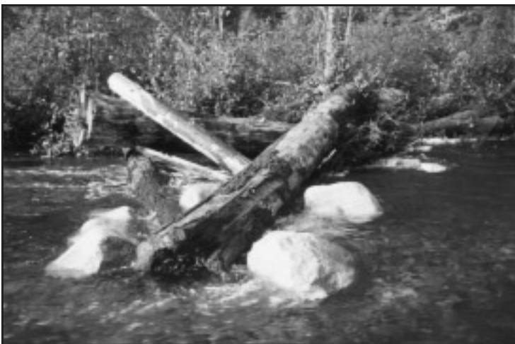
Figure 1. Lateral log jam structure ballasted 2.5 - fold to account for debris collection before scour.
