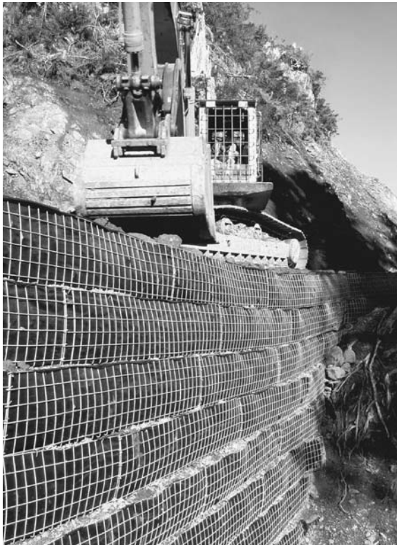
Figure 2. Wire forms are set slightly inwards from the row below.
