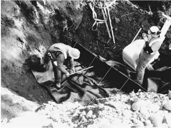
Figure 1. A piece of geotextile fabric is laid on the compacted fill.
