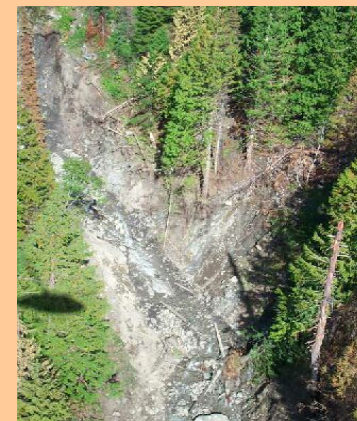
Debris Flow Track
